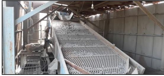
Fig 3.1 Crushing of demolished waste in a crusher
