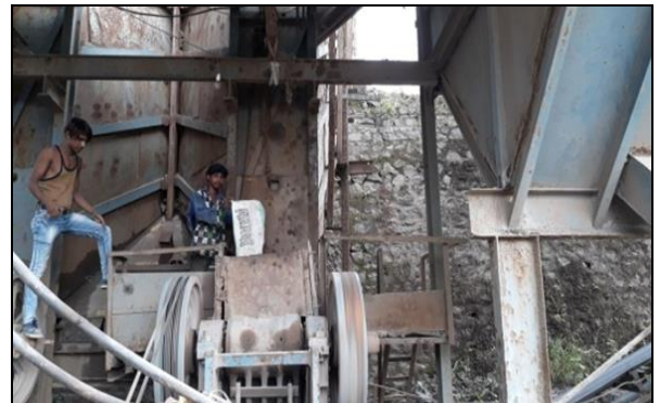
Fig 1.8 Jaw crusher to crush the demolished waste
