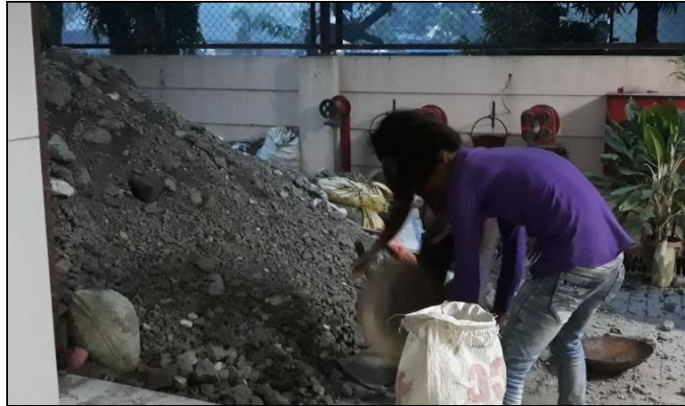
Fig 1.7 Demolished waste collected from site
