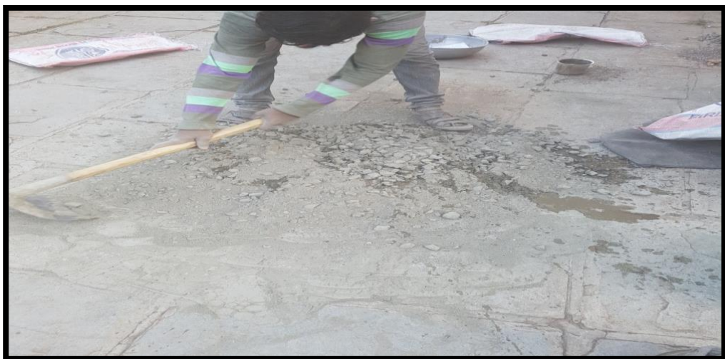
Figure No 5.6 MIXING OF CONCRETE INGREDIENTS
