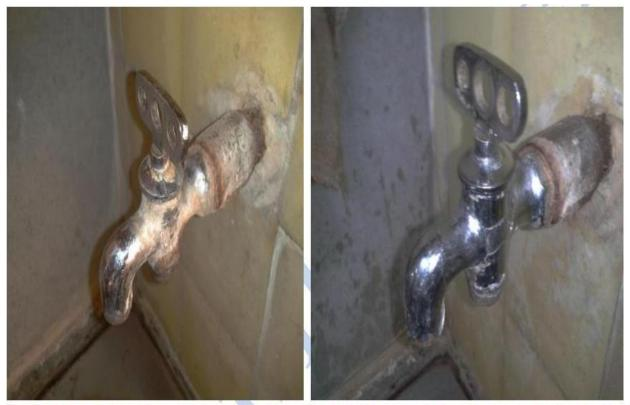
Due to hard water often these scaling happened (1st Image) in bathroom or home appliances. 2<sup>nd</sup> image is the result from water conditioner without using any chemicals.
